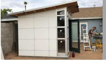
FASTENERS: 1 1/2" 16 Gauge Brad Nails (Hardie Siding) 3/4" 18 Gauge Brad Nails (Metal trim) Decorative Screws & Washers
